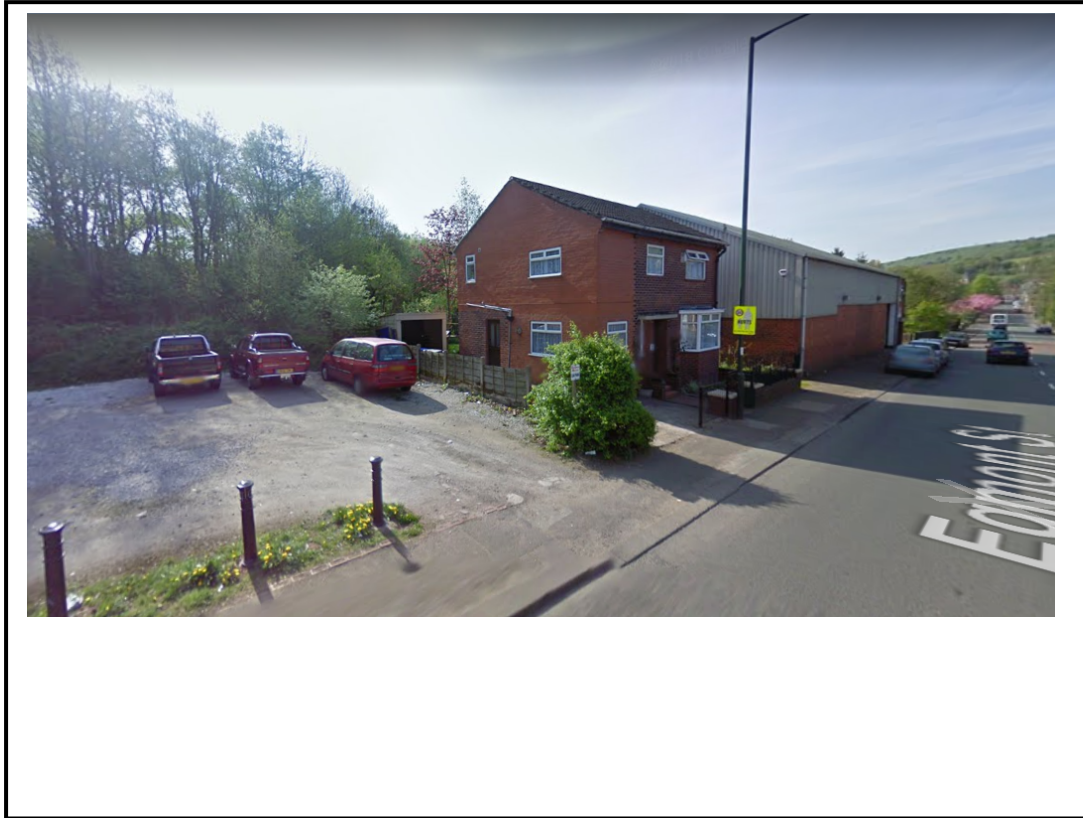
Photo 5 – view of the existing building and neighbouring property at 60 Egmont Street, which is adjacent to the north eastern corner of the application site.
